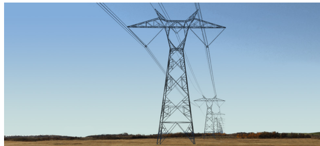
Photo simulation of towers for the 500kV Eastern Alberta DC Transmission Line
