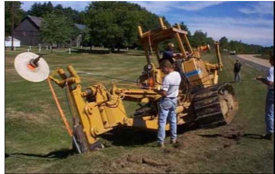
Installation of fibre optic cable
